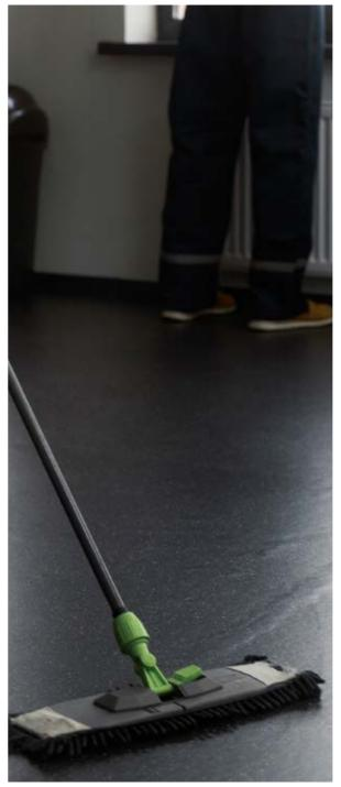
After laying the material it is essential to clean them thoroughly. If residues of grouting are not removed properly or quickly, this may result in stains that are difficult to remove and may create a film of concrete on the floor that traps all kinds of dirt.
